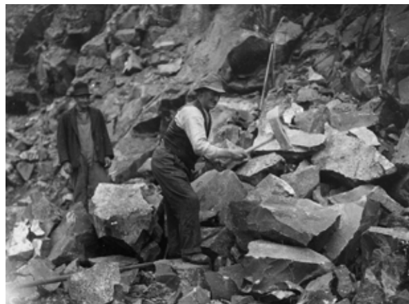
Rock being broken by hand © Belfast Telegraph Collection Ulster Folk and Transport Museum (Ref: HOYFM.BT.0948)
