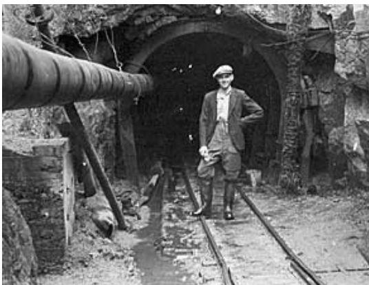
Sam McMurray, the Contractor's Engineer, at an entrance to the Binnian Tunnel (1950) Courtesy of Mr Norman Ervine
