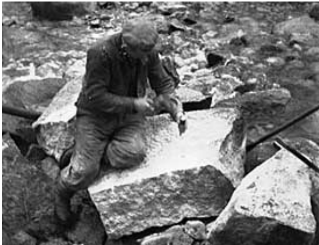
A stoneworker splitting granite by hand using the plug and feather technique Courtesy of Mr Norman Ervine
